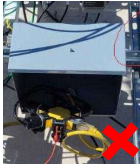
Disordered wiring of distribution box
