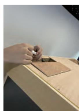
14. To install the handle of the sauna door, first remove the handle from the top inner power box, and then remove the screw, from the door to the outside, pay attention to put the round plastic pad into the glass hole, the screw tip comes out a little, and finally align the screw hole of the outer handle, and tighten the screw.
