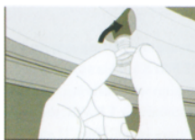
a. Screw in the anti-theft nut first
