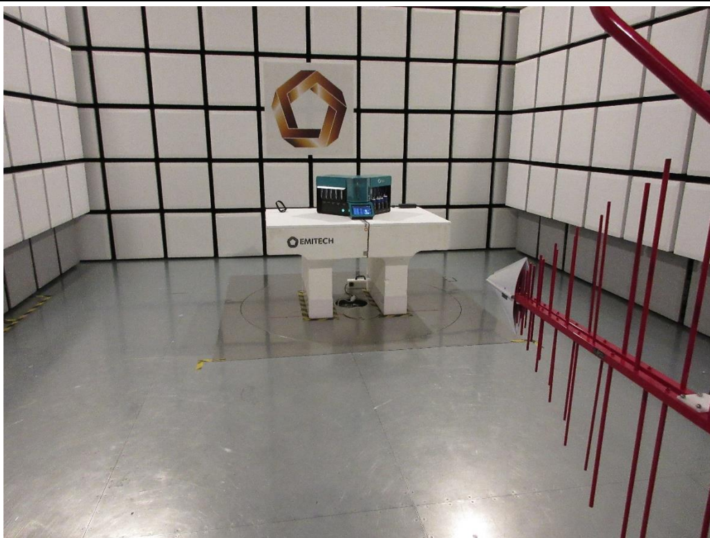
TEST SETUP PHOTO(S) - CISPR 11
