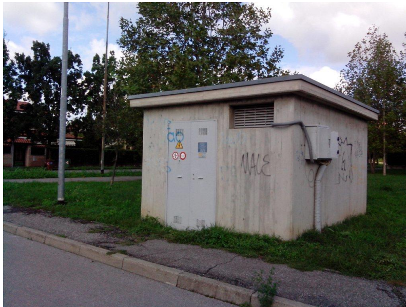
Figure 2 - Pre-assembled substations
