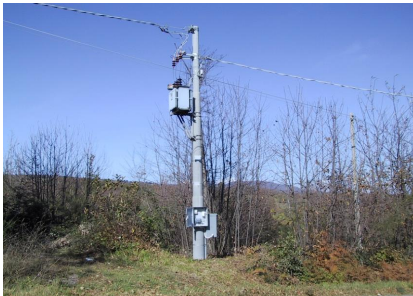
Figure 3 Pole-mounted transformer
