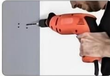
Step 2: Make 4 small holes in the wall
