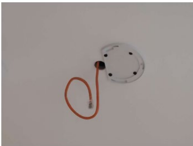
Intelligent gateway base installation signal
