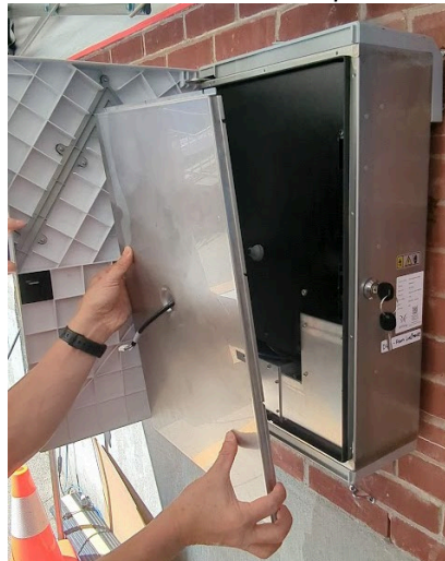
Figure 10: Removing the metal shield
