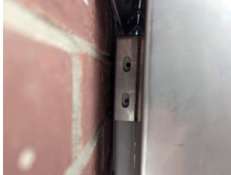
Figure 5: Wall Box Secured to Wall
