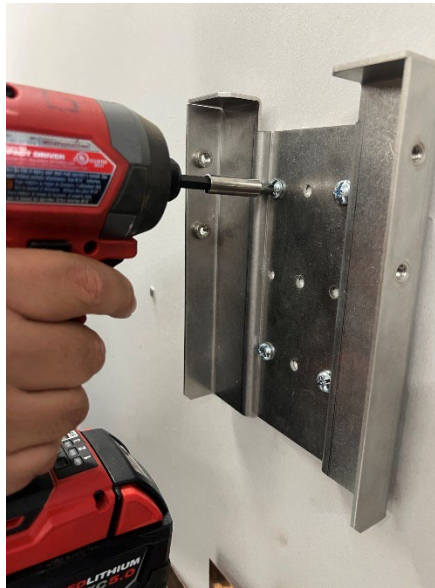
Figure 3: Driving screws into wall through bracket
