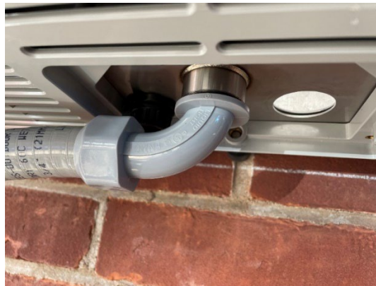
Figure 13: Liquid Tight Elbow
