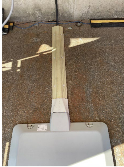
Figure 28: Ground Pad Assembled with Ground Conduit
