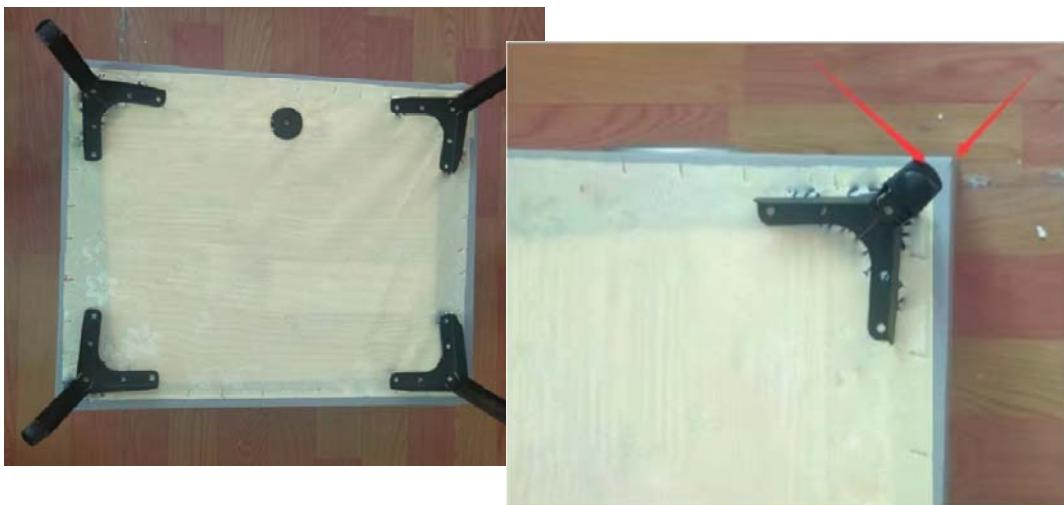
The corners of the feet are aligned with the corners of the cabinet when viewed from the front
