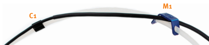
Figure 11. Place the first marker (M1) on the heat shrink tube and the first clip (C1) after the heat shrink tube. (The photograph is showing a close-up of M1 and C1 in Figure 10.)
