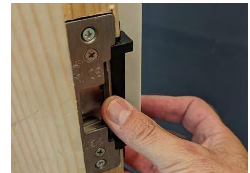
Try again. This time after it beeps, push the electric strike with your finger to check that it has released. After 5 seconds it should lock back in place.
