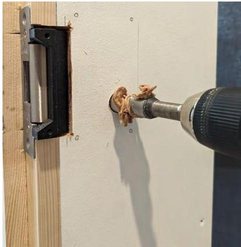
5. Mark up the position of the cable and mounting screws and drill a  $\frac{3}{4}$ " (19mm) cable hole.
