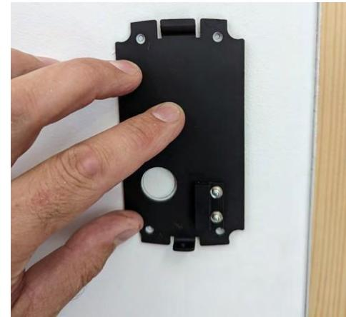
8. Position the keypad backplate and mark the position of the cable and fixing holes.
