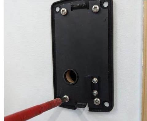
**12. In this instance we will use the rubber gasket.** Place the gasket over the pre-drilled holes and then align the backplate over the gasket. Fix to the wall using the 4 included fixing screws.
