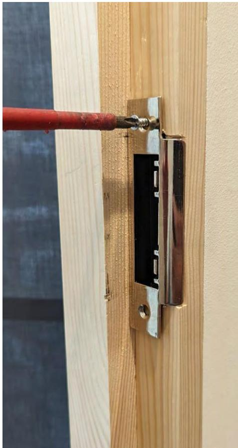
**1. Remove the existing strike plate from the door frame.**
