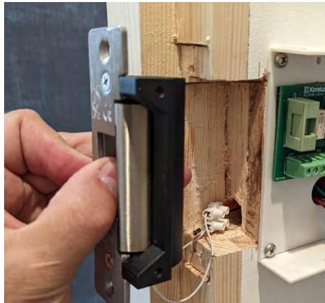
**17. Refit the electric strike and carefully feed the cables through the door frame.**
