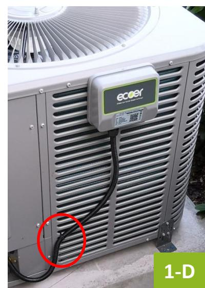
2. Unscrew the cable locker cap and securely fasten the **waterproof joint** to the reserved hole (plug has to be removed).
