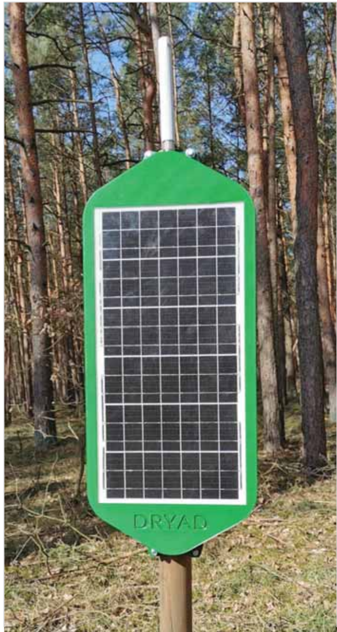
Mesh Gateway deployed on pole
