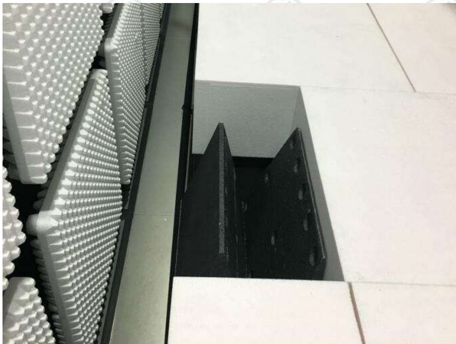
There are absorbing materials under the ground
