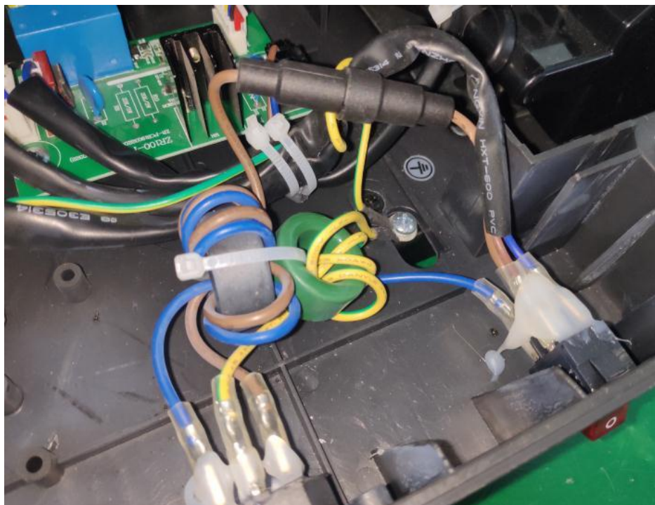
Earthing connection on the metal frame
