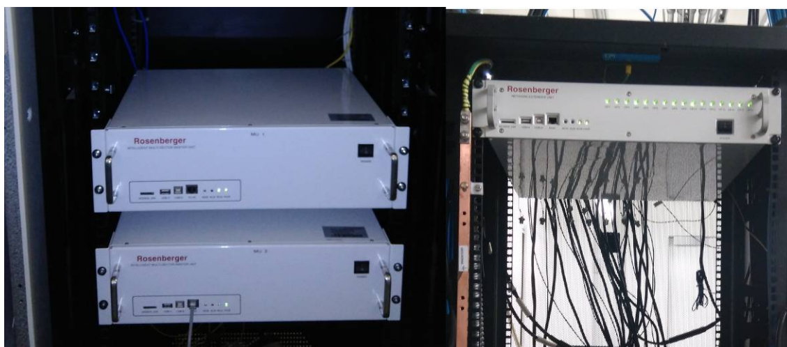
Figure 17 Installation of IM2U and NEU
