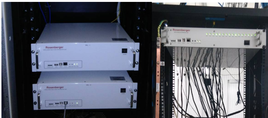
Figure 17 Installation of IM2U and NEU
