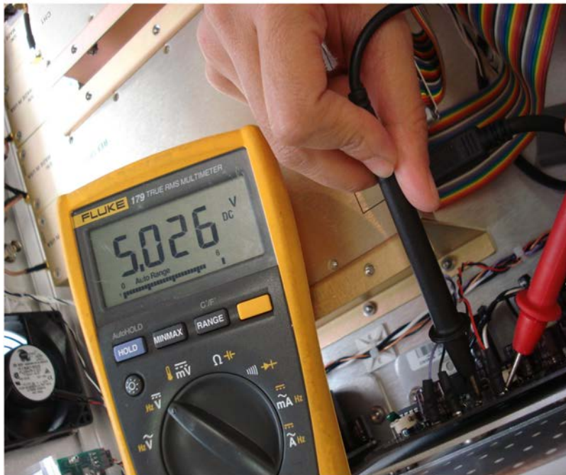
+5V supply in the receiver chassis.
