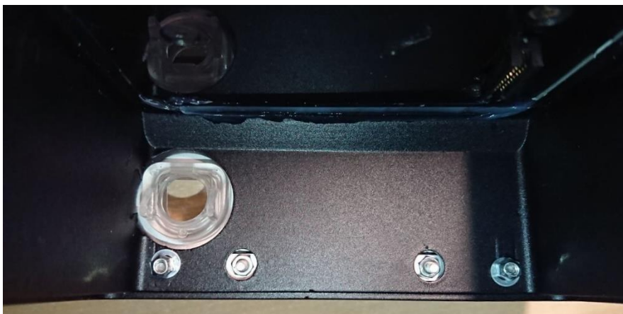
Internal view of the boards assembly place
