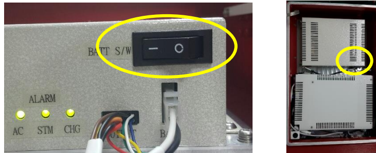
Figure 2 - 8 Battery Switch
