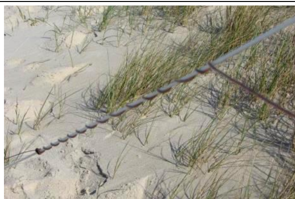
Radials twisted around guide rope
