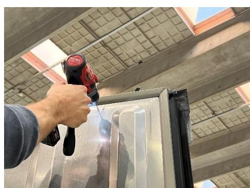
10. Use a screwdriver and 2 screws to mount the magnet. If using glue, press the magnet firmly into position and hold it there for 1 minute before applying some tape to hold it in place while the glue is drying. Leave the container door open.
