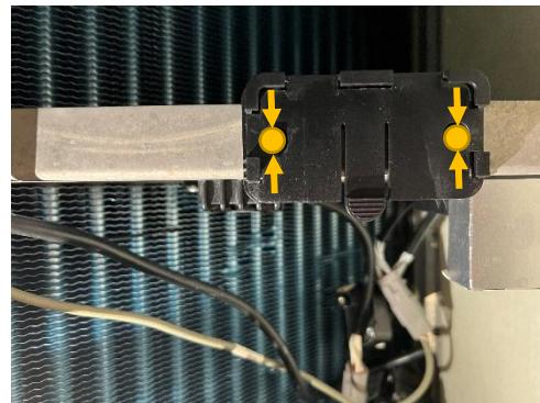
13. Using a drill size 3.8 – 4.0 mm, make the 2 holes.
