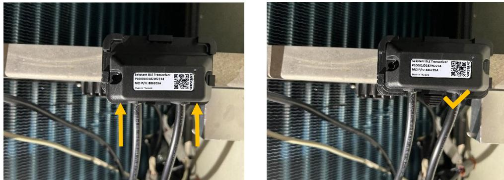
16. Disconnect the humidity sensor from the communication cable and connect the transceiver to the communication cable and the humidity sensor.
