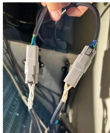
17. Secure the cables with cable ties if necessary. The cables must **not** hang down touching the evaporator fins.
