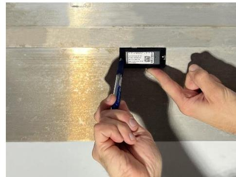
6. If using screws, drill 2 holes size 3.8 - 4.0 mm. Otherwise apply Sikaflex 295 glue to the back of the sensor.
