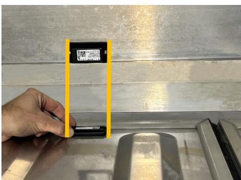
9. If using screws, drill 2 holes size 3.8 - 4.0 mm. Otherwise apply Sikaflex 295 glue to the back of the magnet.
