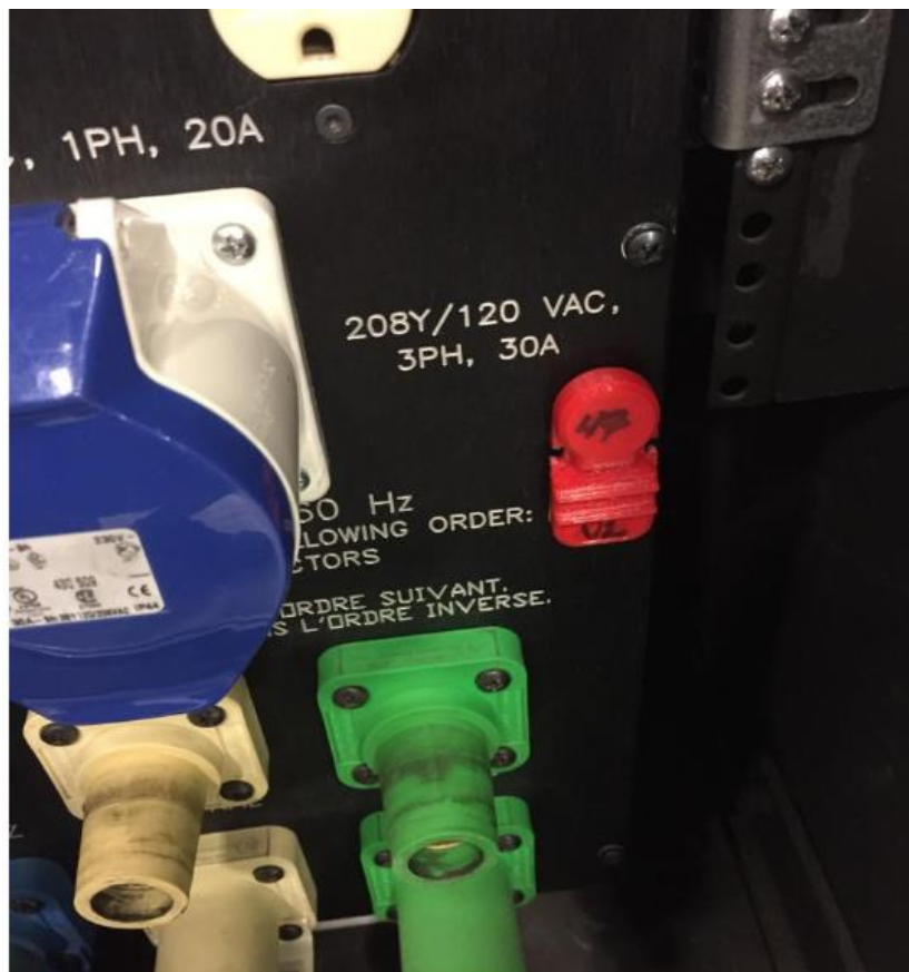
Sample Tag surface mounted with VHB tape (3M5952)
