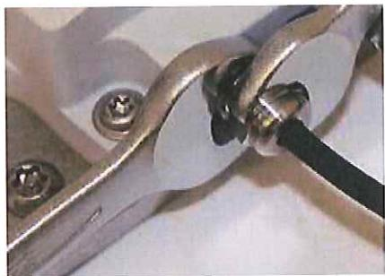
The tightening torque is 6 Nm. You can check this with the help of a suitable torque wrench to be certain:
