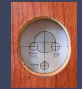
matching the backset for your door. Place the template on the door and position. If a 2 1/8" boring hole already exists, ensure the template matches the existing hole by viewing from the other side of the door.
