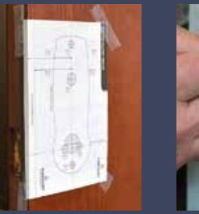
Also ensure that the center of latch line on the template is exactly centered over the latch opening on the side of the door. Once template is aligned, tape it to the door.
