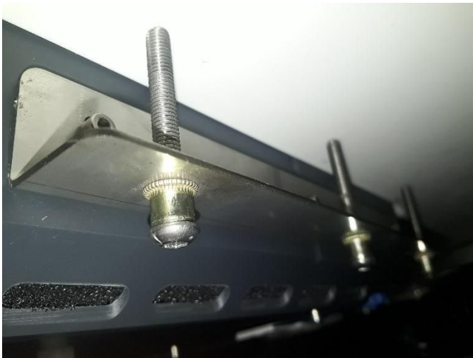
Screws tightened to secure unit below countertop
