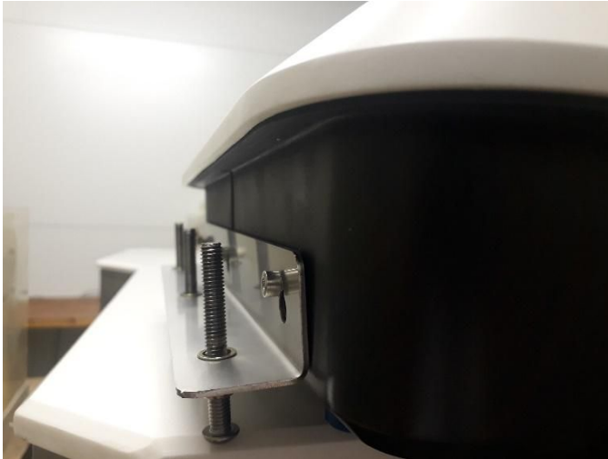
Assembly before dropping into countertop cut-out
