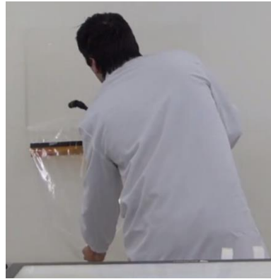
Fig.14 Pull the protection layer and apply soapy water until removing it completely.
