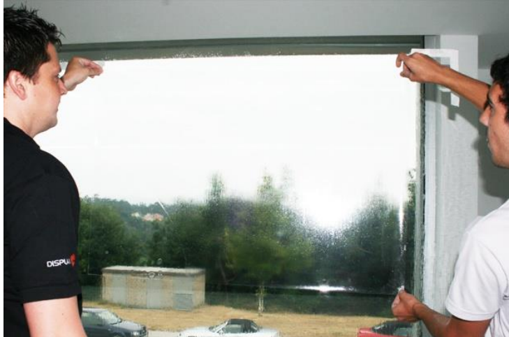
Fig.2 Place the "Cling" against the glass, previously wet with soapy water, where we want to laminate the Touch Sensor
