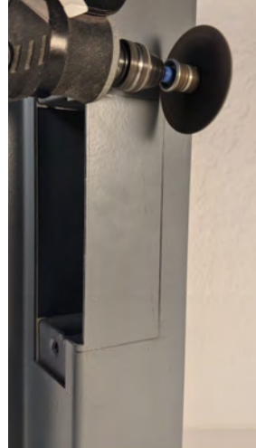
Cut Front of Frame
