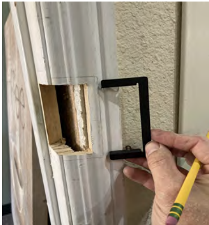
Due to Trim on door, mark and cutout for trim enhancer
