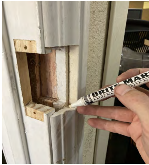
If possible, add paint with valve paint marker
