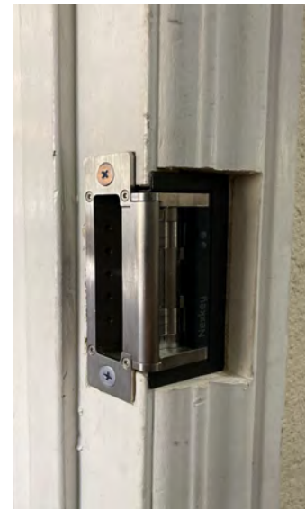
Secure Lock and Test (Shim Strike towards lock if needed)
