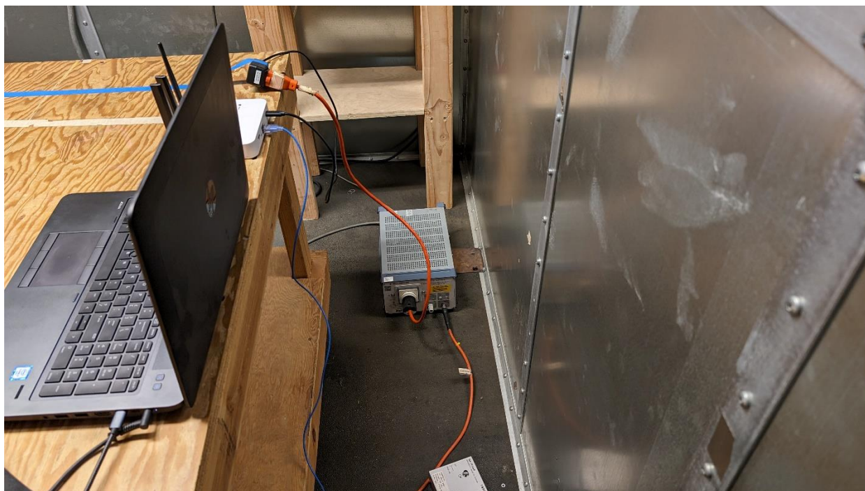
AC Wireline 120VAC Side
