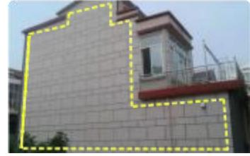
Attention: There must be a solid wall between the indoor antenna and the outdoor antenna to prevent self-oscillation.
