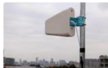
Step 2: Connect the outdoor antenna to the BTS port via the cable and tighten the connectors at both ends, make the outdoor antenna point to the base station
