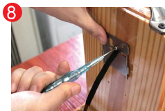
Tighten screw to fix steel board.
