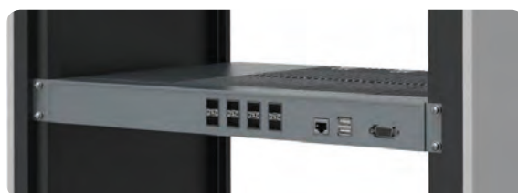
Fig. 10: Place C-hub in rack
