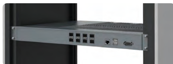
Fig. 10: Place C-hub in rack
