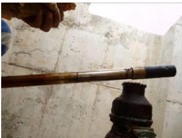
Figure 41: Maintenance of a flow meter measuring water loaded with metal particles
