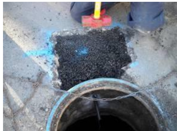
Figure 40 : Aerial buried under asphalt
