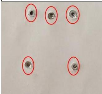
5. Use self-tapping screw TA4\*30 to fix the base.
