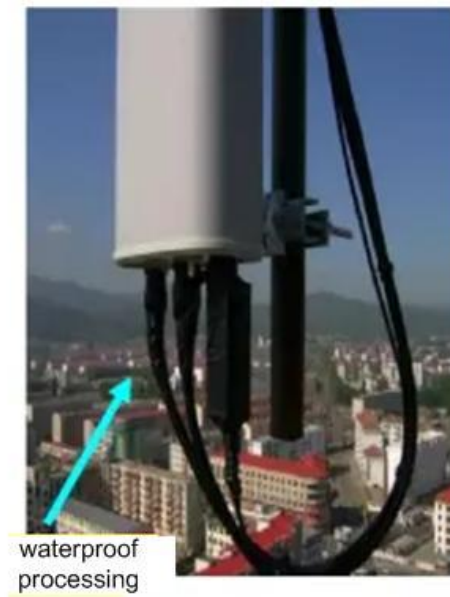
Figure 3-13 Antenna Waterproof Protection
