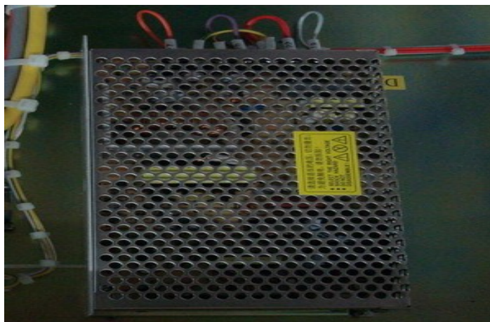
Power unit for emergency starting up
