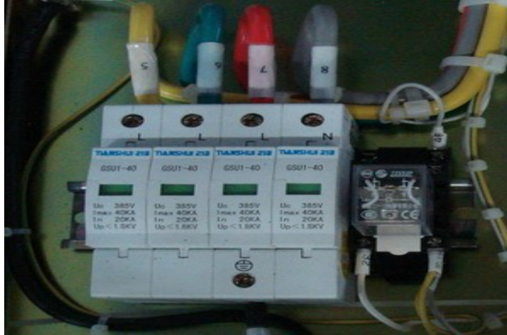
Lightning arrester on power distribution unit
