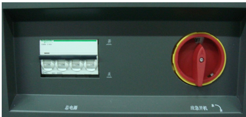
Air switch and emergency switch on the power distribution unit
