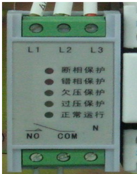
Phase dislocation and phase lack protection unit
