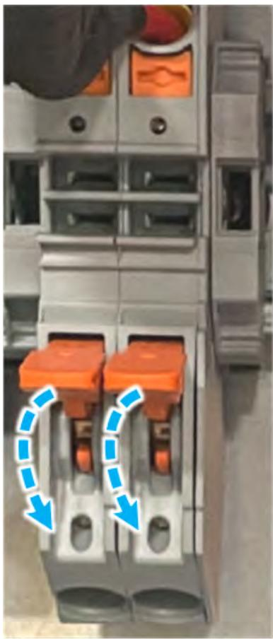
*Press down the levers to engage the connectors.*
