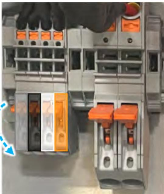
*Press down the levers to engage the connectors.*
