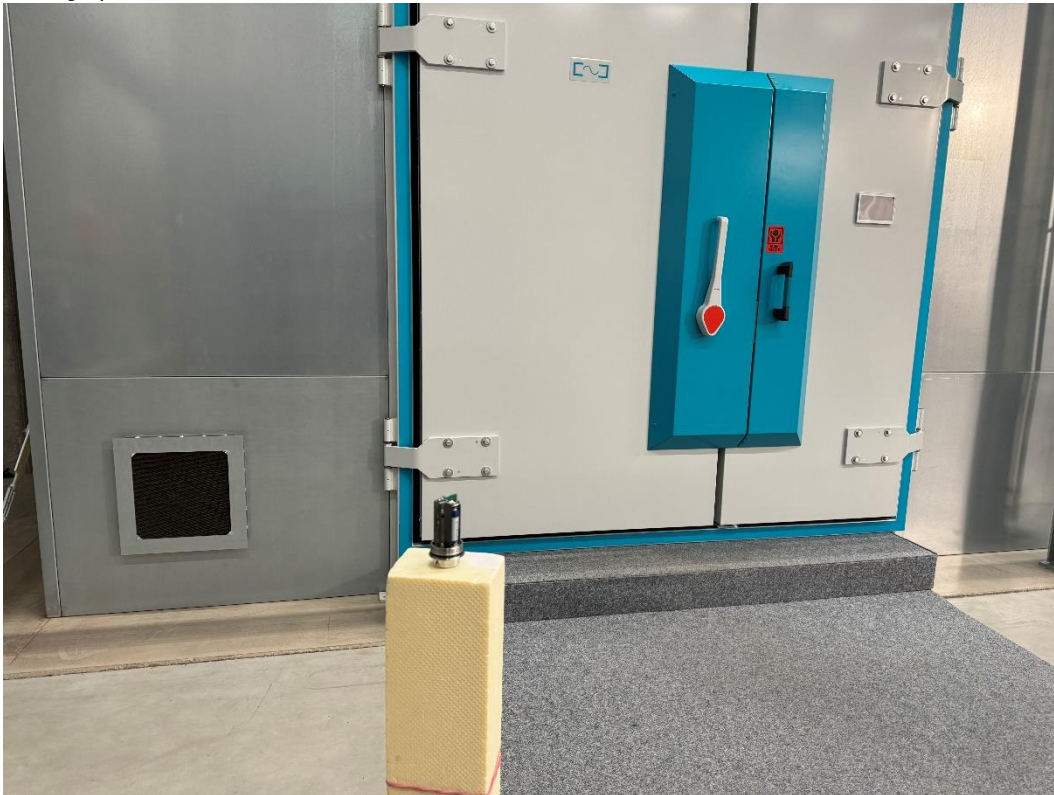
Photograph 15: Overall view 2, door closed.
