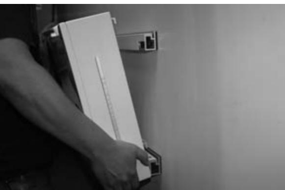
17 Connect AC cable provided to back panel of Habitat1. Lift cabinet to wall and lower onto brackets.
