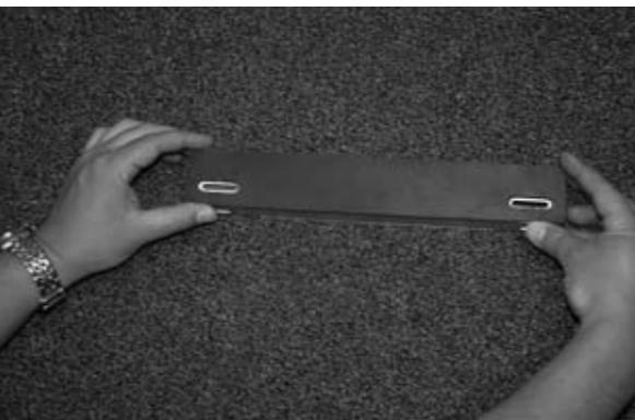
15 Place short gasket on the back side of wall bracket C. Gasket **must** go between wall and bracket. *Do not omit the use of this gasket.*
