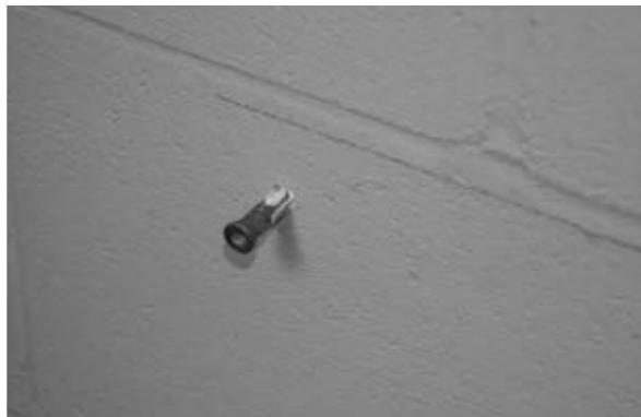
10 Push masonry anchor into wall and drive flush with hammer.
