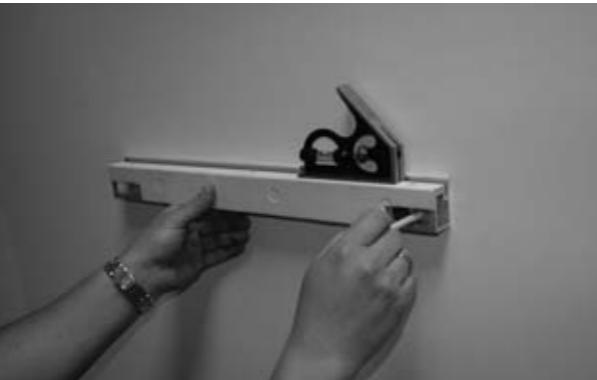
7 Level the bracket against the wall and mark the screw hole locations. Make sure that the screws will hit the studs.
