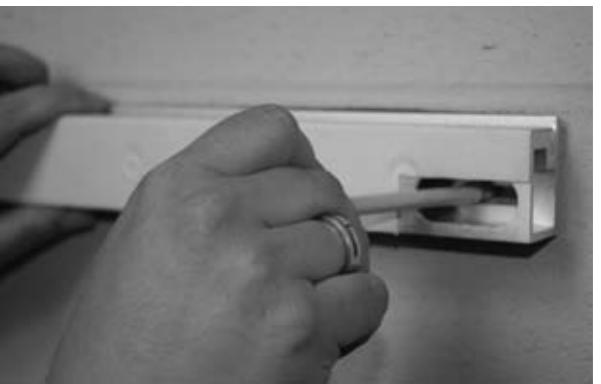
6 Level the bracket against the wall and mark the screw hole locations.
