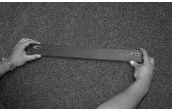
9 Place long gasket on the back side bracket A. Gasket **must** go between wall and bracket. *Do not omit the use of this gasket.*
