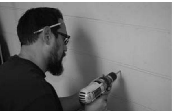
8 Drill hole for anchors using the drill / driver and 5/16 inch drill bit.
