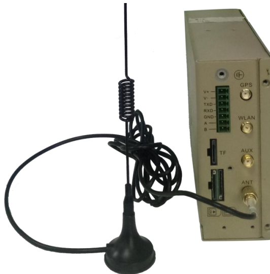
Figure 3-6 Installing an Antenna
