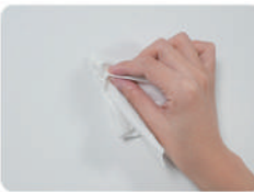
Clean the wall before installation
