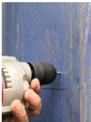
Figure 2-5 Drilling of Mounting Bracket
