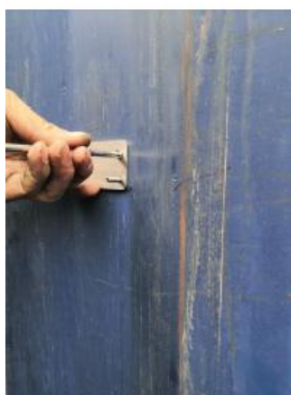
Figure 2-6a Fixation of Mounting Bracket
