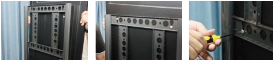
Step 6 : Hang the screen on the stand (pay attention to the positions in the figure) .
