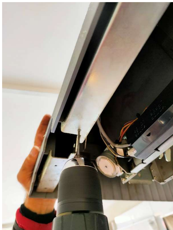
4. Drill 2 x 3 mm holes for both locks
